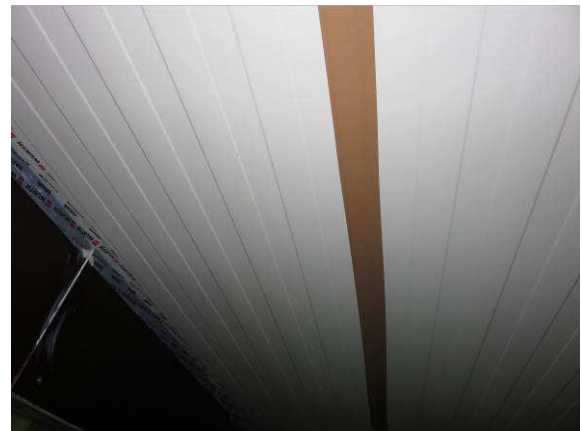
Photo 3 Covering internal joints for zero measurement
