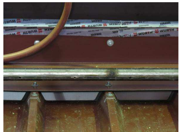
Photo 5 Water line for surface water
